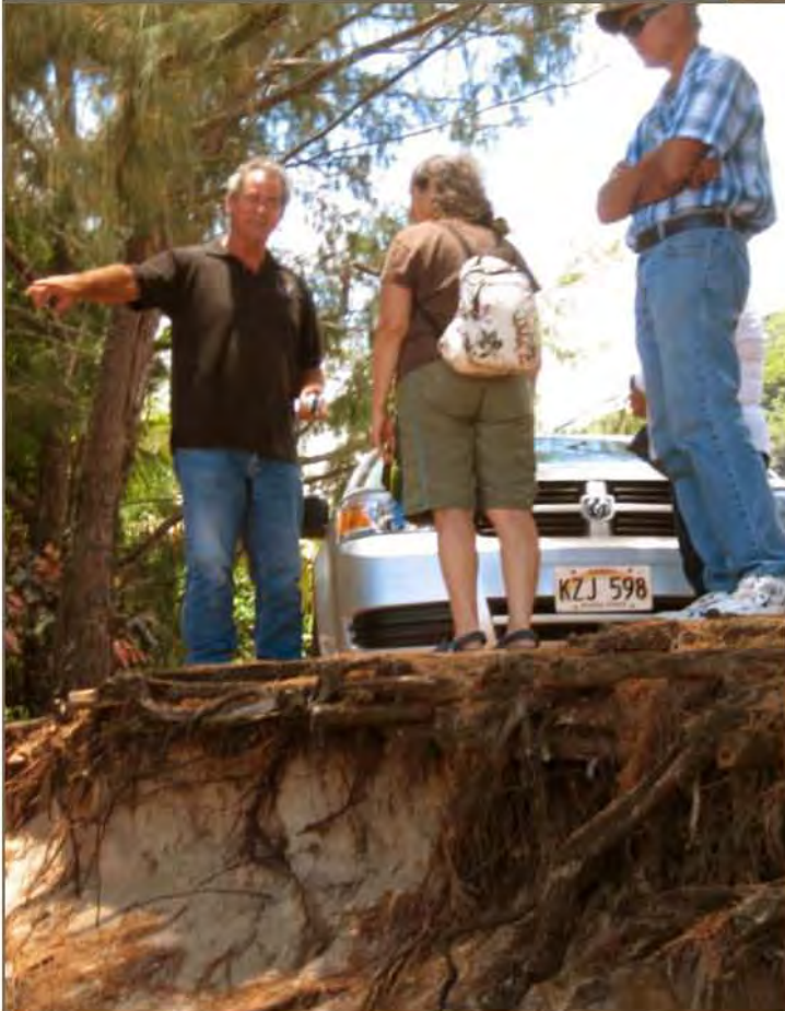
Haena. Shoreline erosion at one of several areas used by public for shoreline access. Parking problems.
