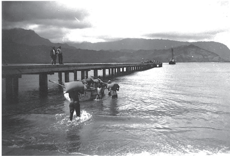
Transporting rice to market at the Hanalei Pier, date unknown. SOURCE: Historic American Engineering Record HI-17.
