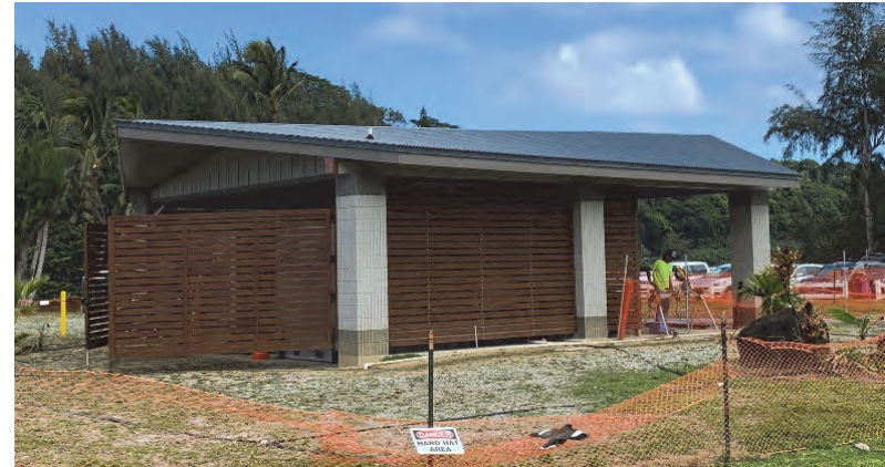
Construction of new comfort station, February 2020.
