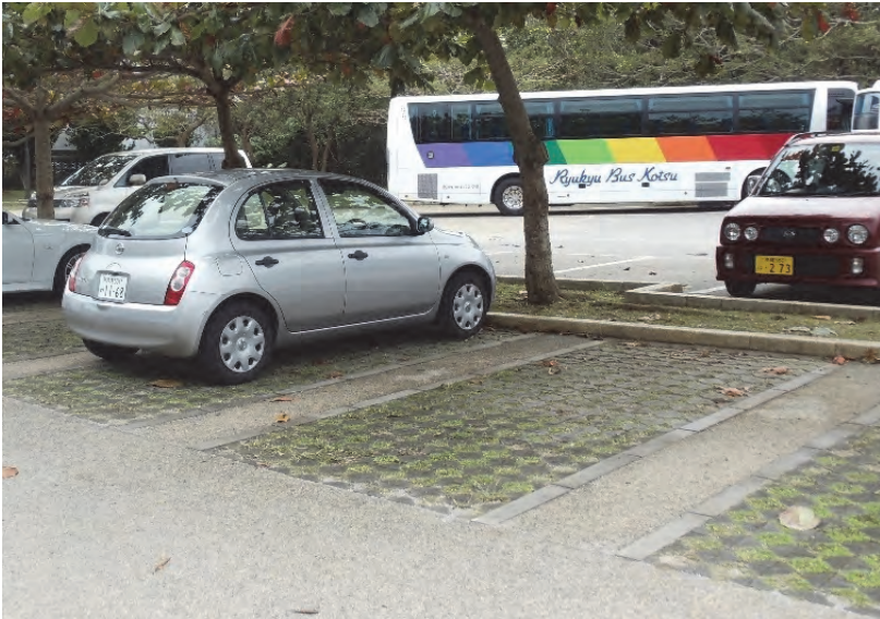
A combination of permeable concrete and pavers used for parking.
