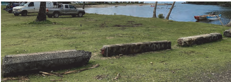
Wooden poles, boulders, vinyl fencing and concrete pilings function as vehicular control barriers.
