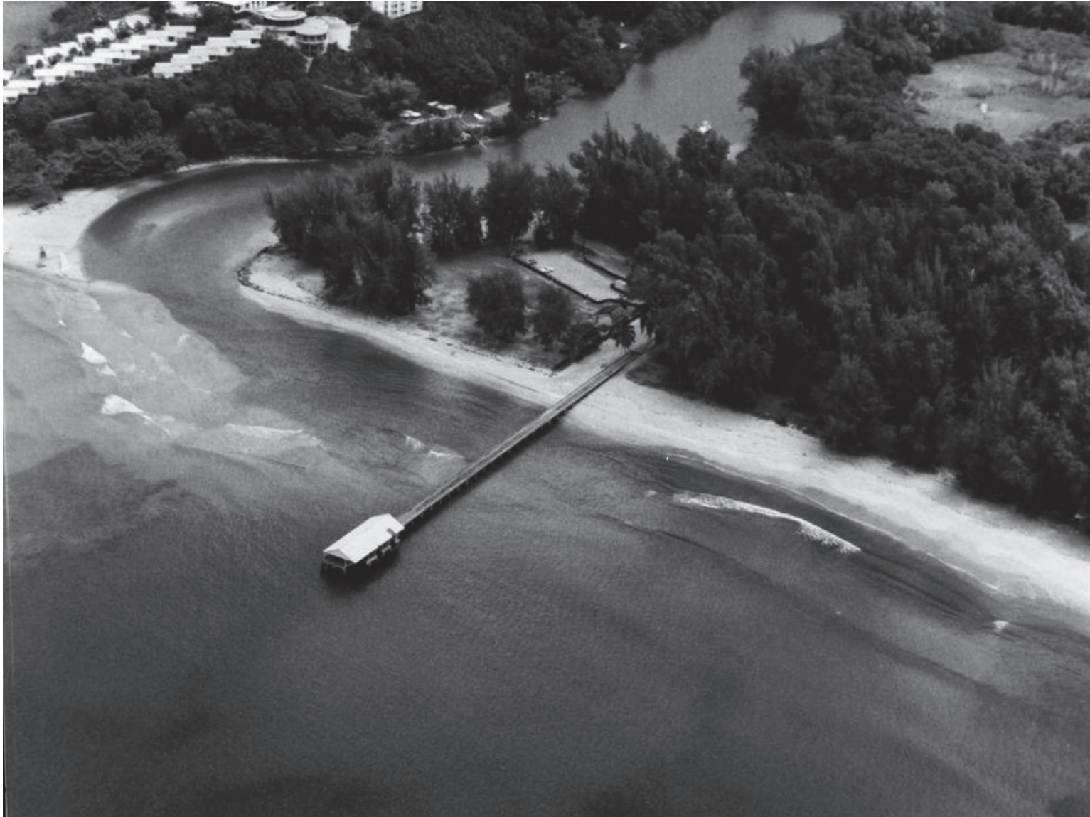
Aerial view of pier and county park, June 20, 1978. SOURCE: Historic American Engineering Record HI-17.
