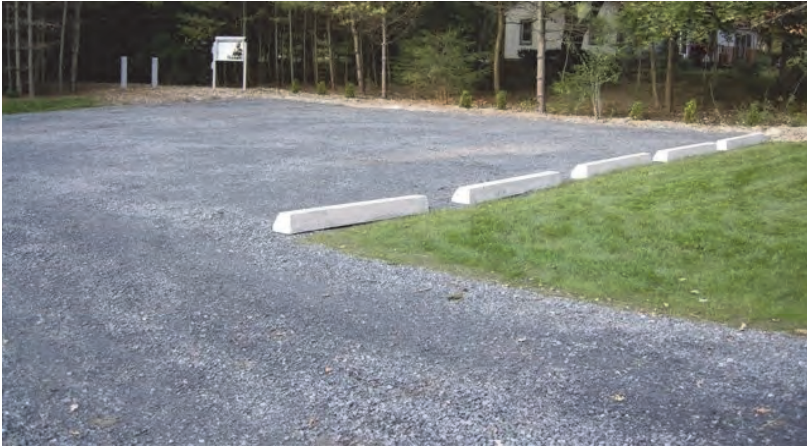
The use of crushed gravel for parking lots reduces surface runoff. Depressed grassed area functions as a drainage swale.
