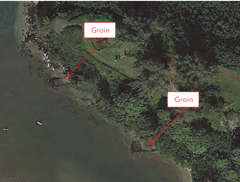
Two small breakwaters were installed on the Hanalei Plantation Hotel side of the river in the 1960s to keep access to the river open for boats during the winter. The hooked shape of the breakwaters was intended to control the current.
