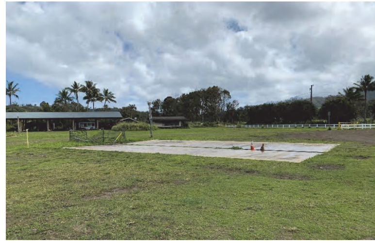
Boat wash pad at Hanalei River Ramp.
