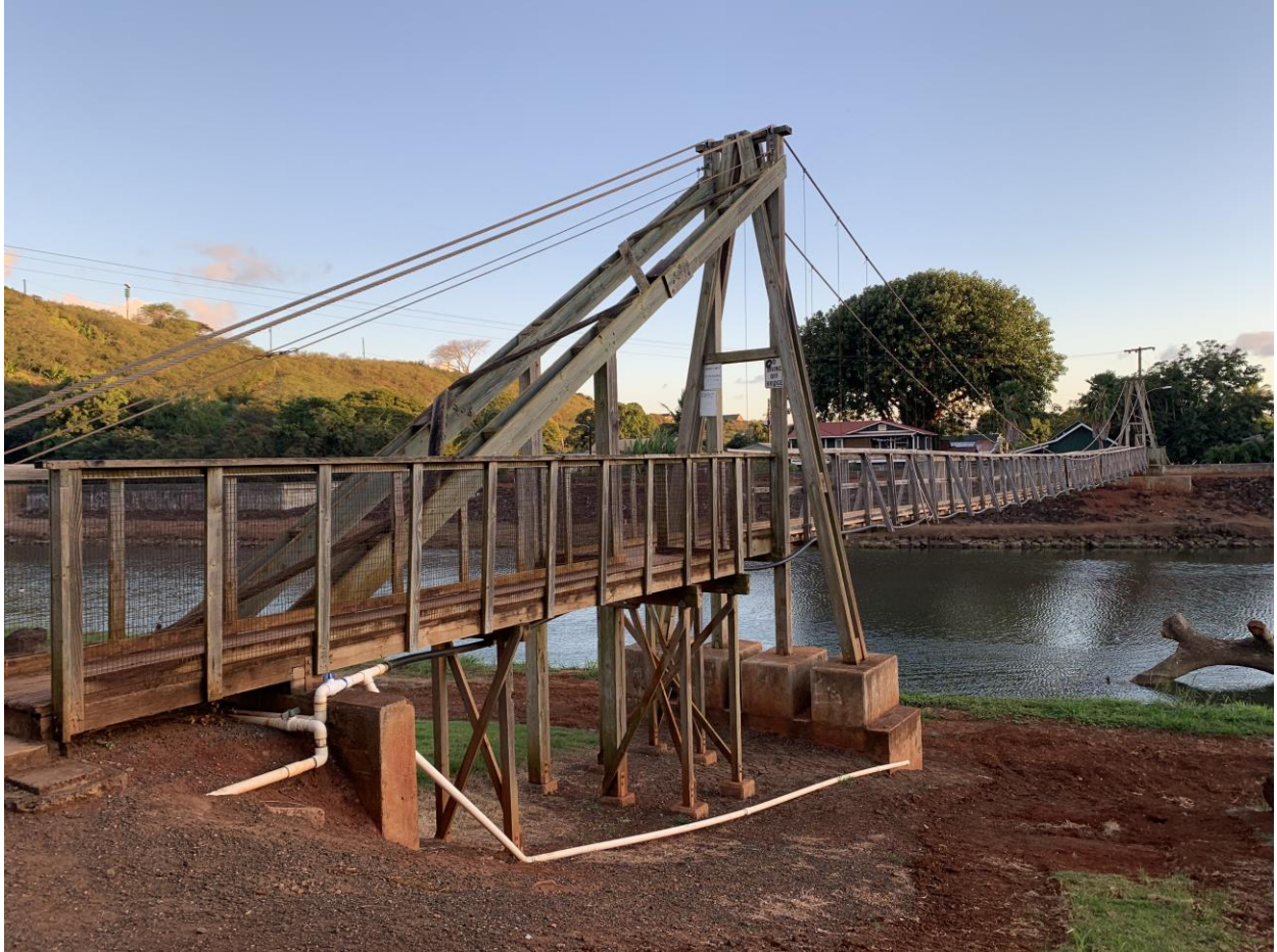
Photo caption: Repairs were completed for the Hanapēpē Swinging Bridge on Feb. 21.
