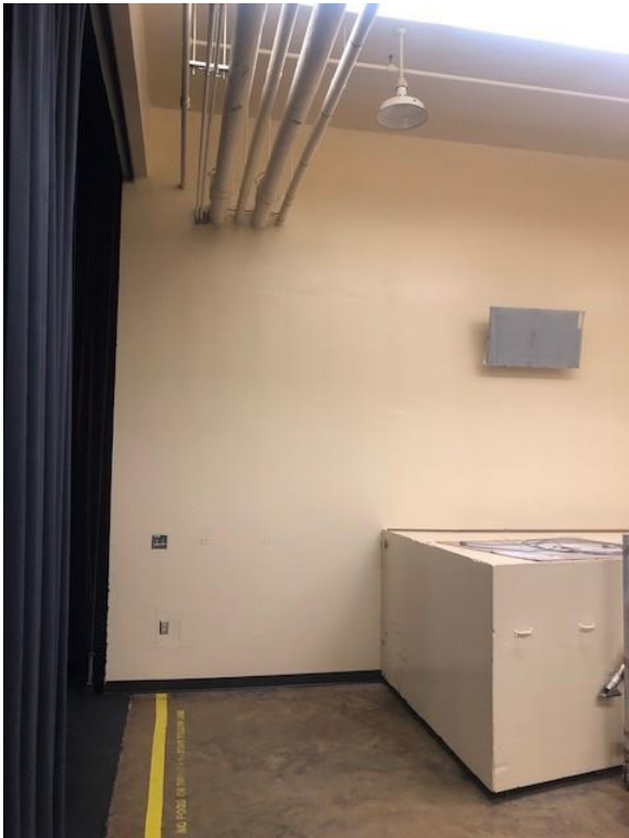
Repainted Stage Right
