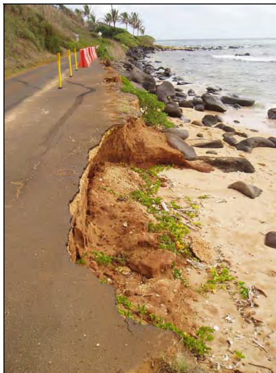
Figure 12. 'Aliomanu Road showing asphalt damage, view to north
