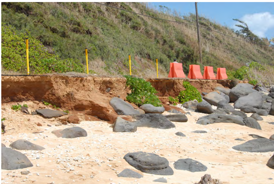
Figure 1-4. Undermining of the road
