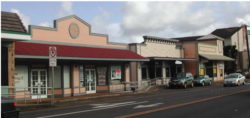
Figure 3-58: New Commercial Buildings on Kūhiō Highway with Western-Style False Fronts
