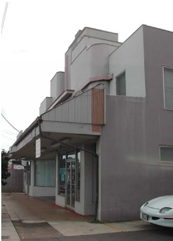
Figure 3-45: Former Theater with Art Deco Details at the Entry on Rice Street
