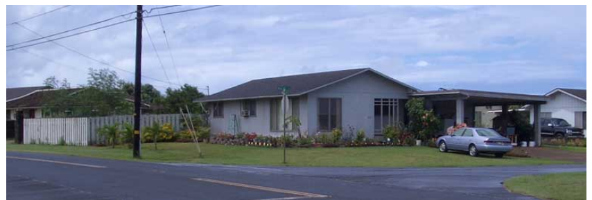
Figure 3-73: Residence on Hardy Street
