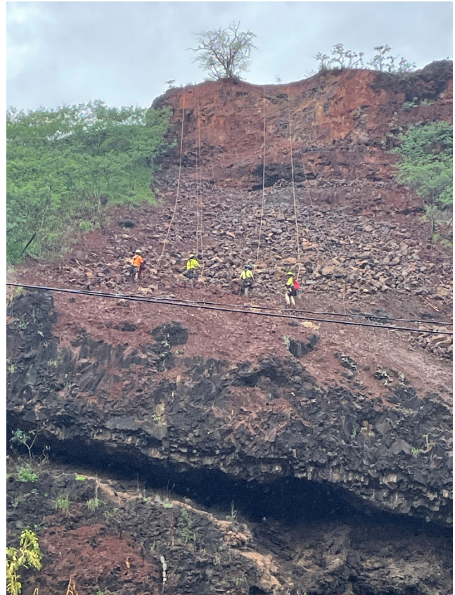
Above photos: The first phase of rock scaling work continued Monday, which includes forcing loose rocks off the slope onto the roadway below.
