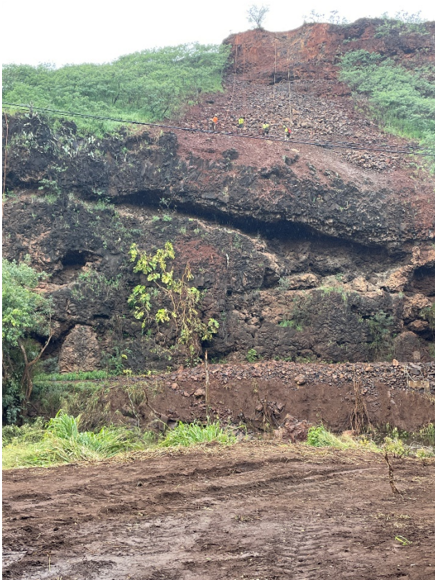
Above photos: The first phase of rock scaling work continued Monday, which includes forcing loose rocks off the slope onto the roadway below.
