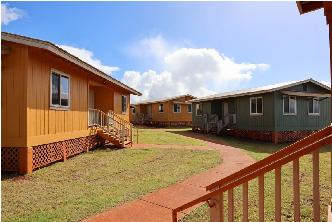
Lima Ola Supportive Housing Project consists of 32 units, studio and one-bedroom, with square footage ranging from 240 to 400 square feet. It also includes a community building with offices, a reception area, and laundry facilities.
