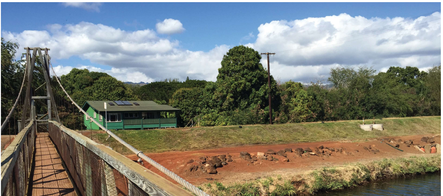
Historic Hanapēpē Swinging Bridge, Hanapēpē-'Ele'ele District
