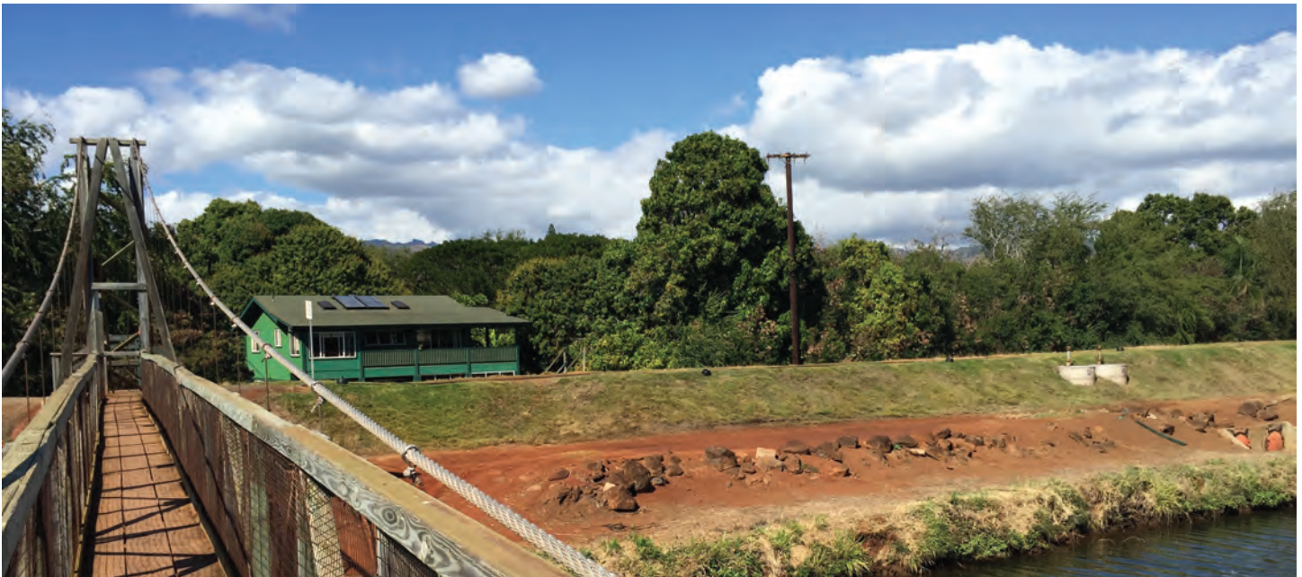
Historic Hanapēpē Swinging Bridge, Hanapēpē-'Ele'ele District
