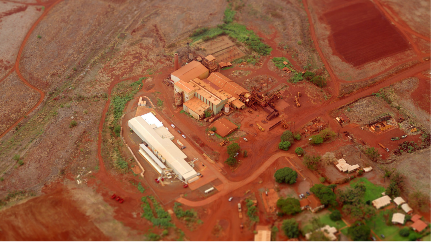
Aerial of Makaweli. Makaweli can accommodate large-scale agricultural activities and has the potential to increase regional food security and generate local jobs.
