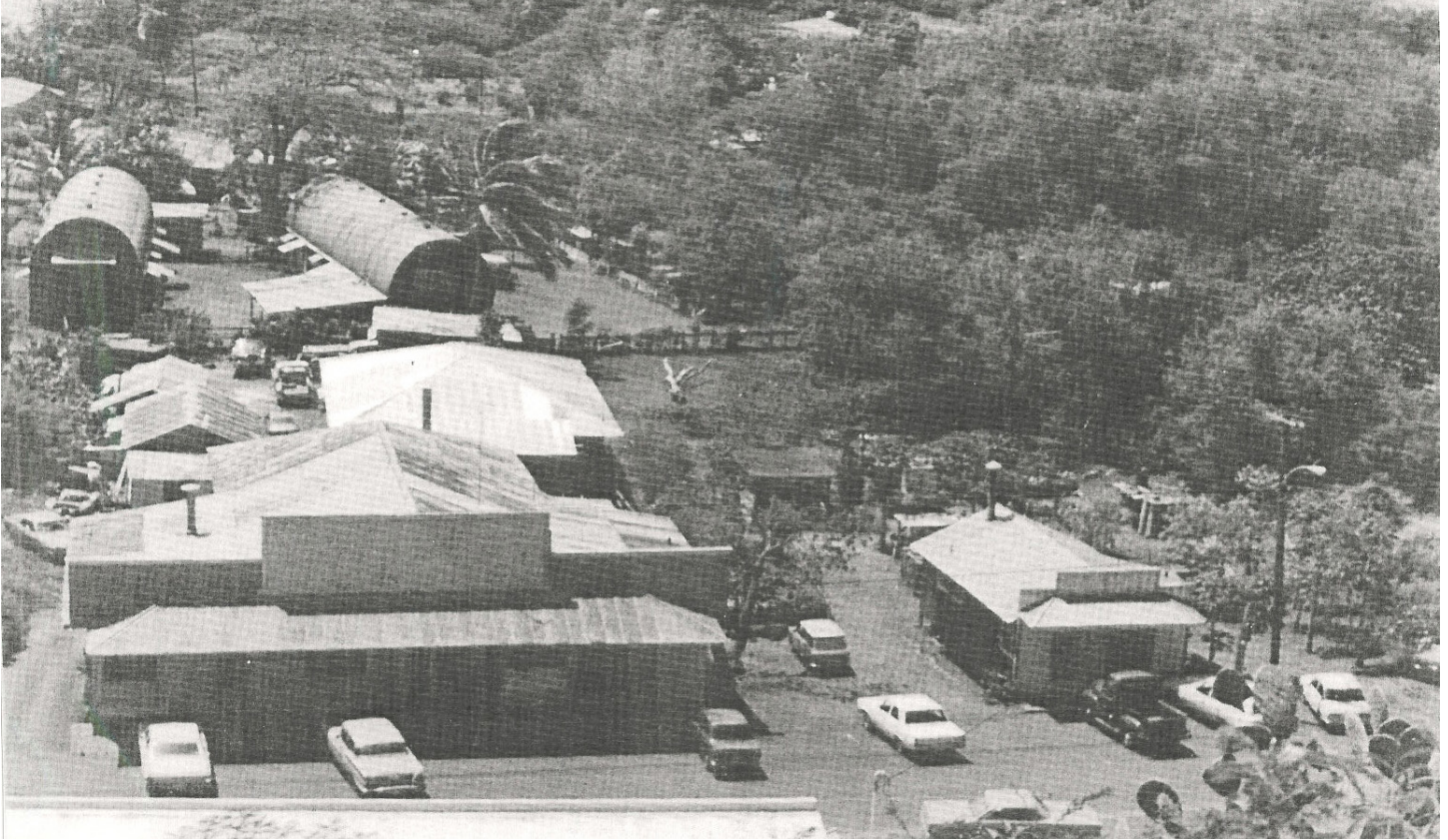
Street-front buildings with quonset huts in rear, Port Allen, 1945. Courtesy of Kaua'i Historic Society.
