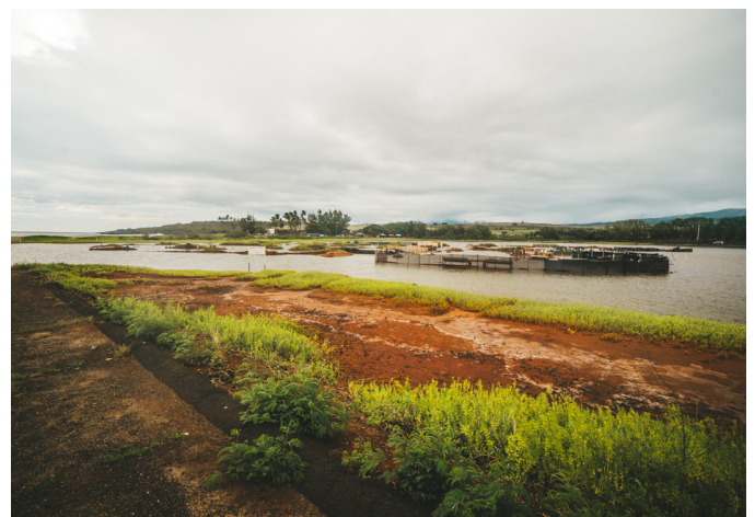
Flooding at Pū'olo Point.
