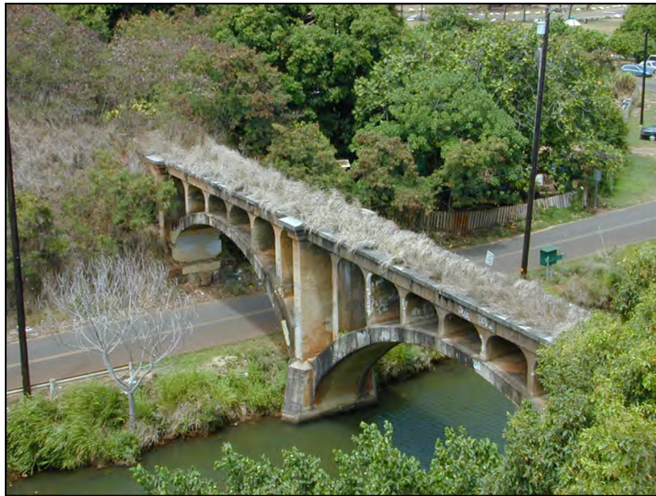
Photo of the Hanama’ulu Railroad Bridge
