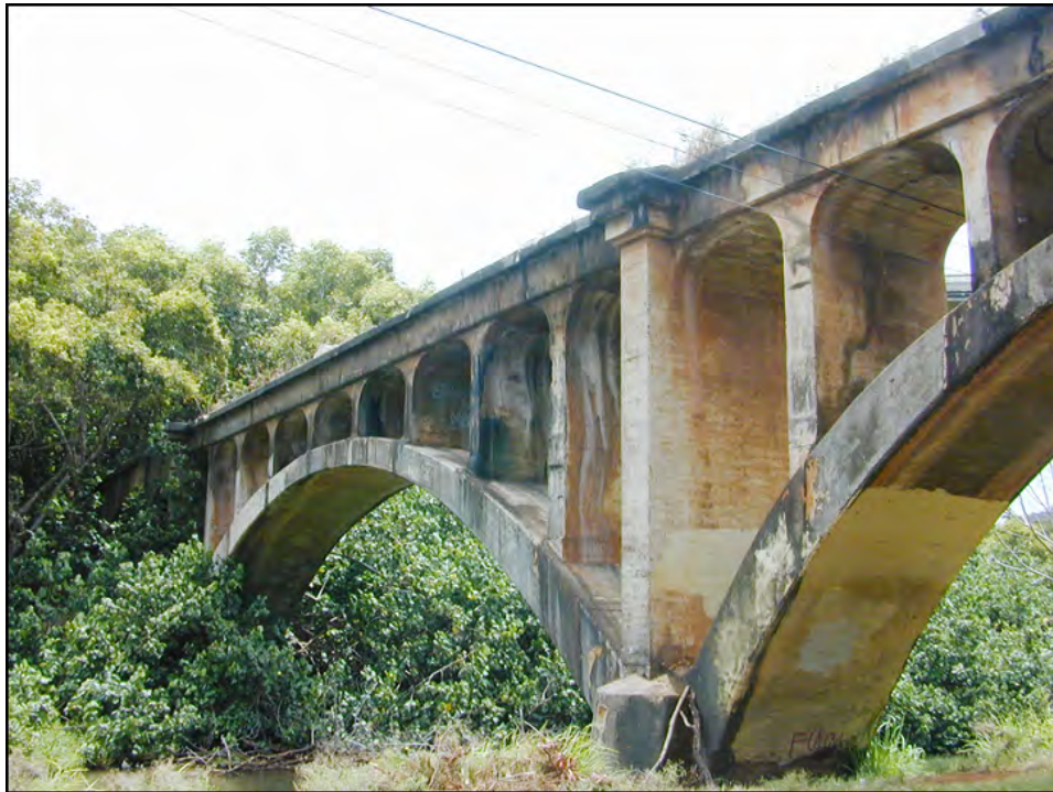
Another view of the Hanama'ulu Railroad Bridge
