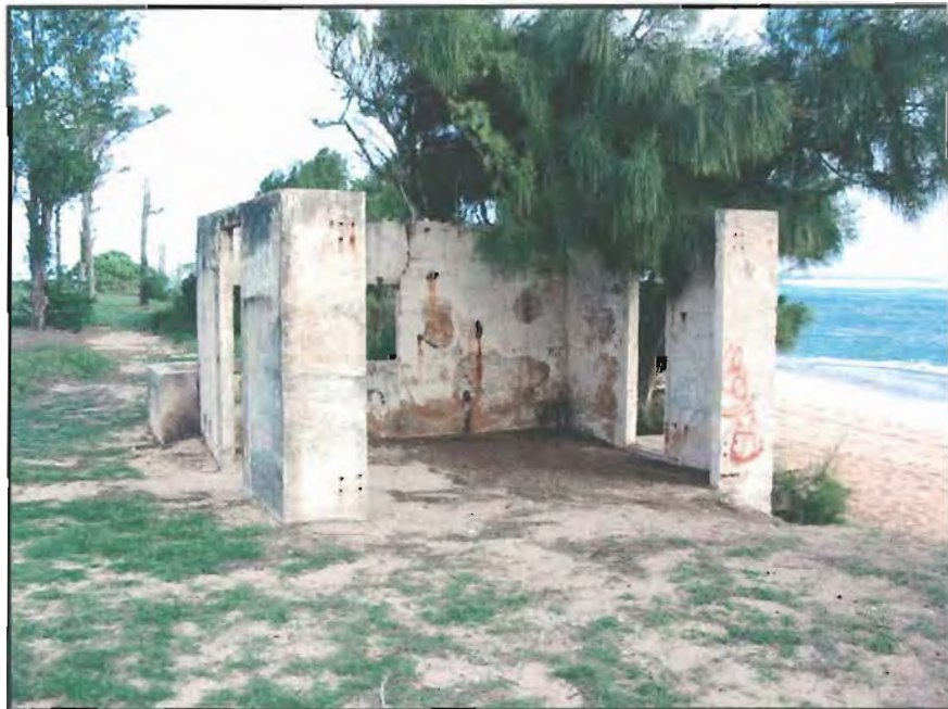
Figure 28: WWII Era bunker located near coastline, view to east
