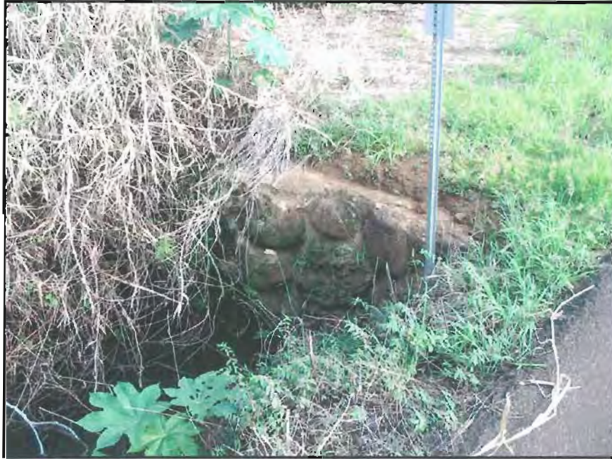
Figure 29: Stone faced railroad culvert, view to east
