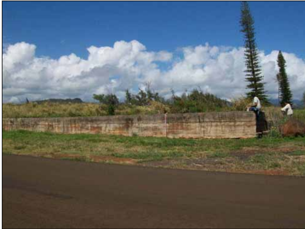
Figure 80. Site 50-30-11-2103 Feature B, roundhouse foundation remnant; view northwest
