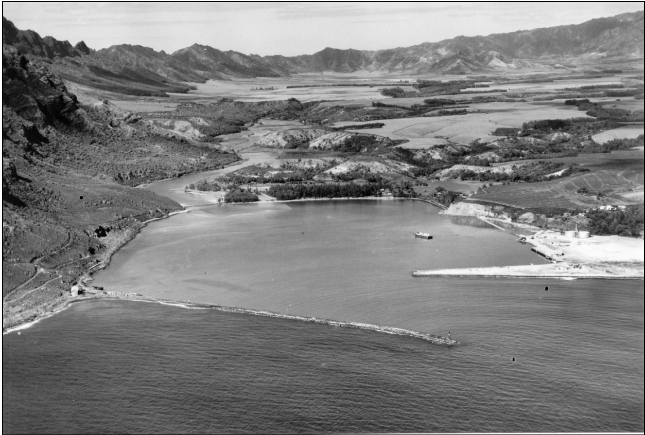
Figure 16. Circa 1930 photograph showing Nāwiliwili Harbor under construction (Bishop Museum Archives)
