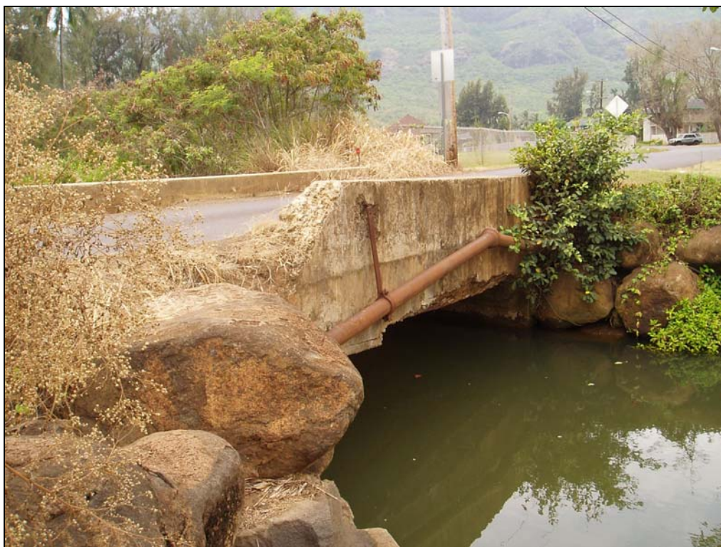
Figure 23. Old bridge spanning Pū'ali Stream, facing north
