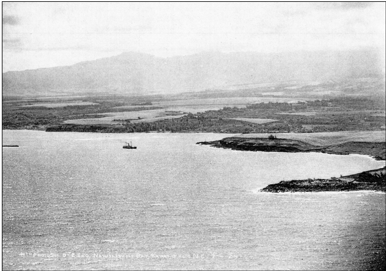
Figure 15. 1924 photograph showing Nāwiliwili Bay before construction of the harbor facility on the north side of the bay (Bishop Museum Archives)
