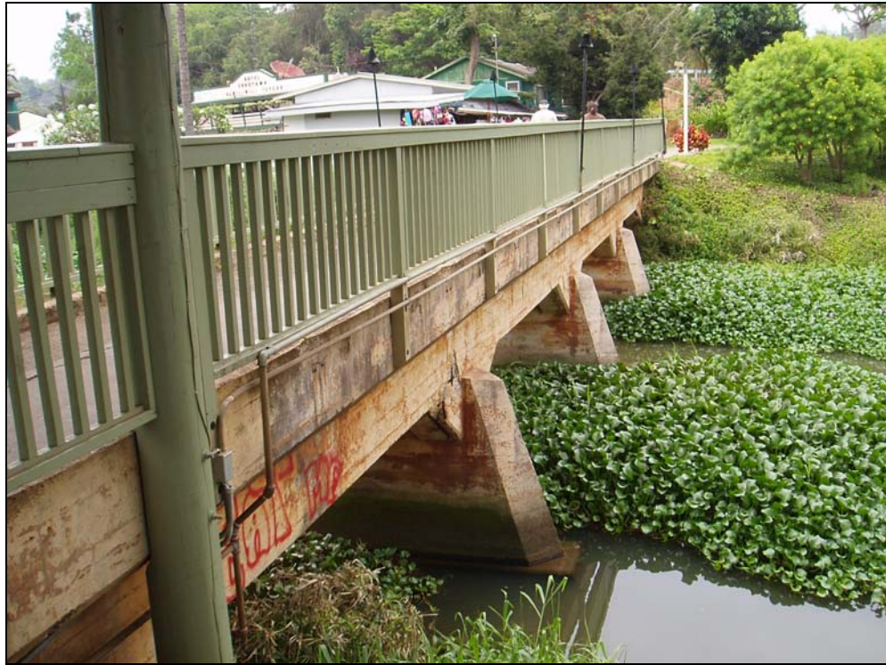
Figure 24. Old railroad bridge spanning Nāwiliwili Stream, facing north
