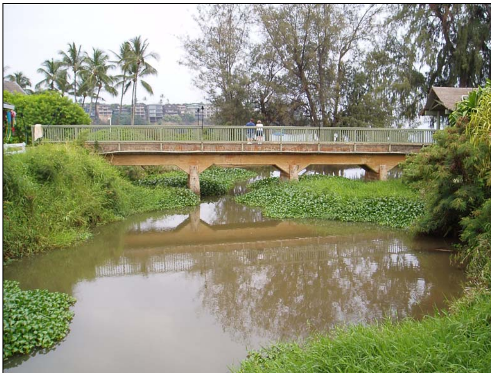
Figure 25. Old railroad bridge spanning Nāwiliwili Stream, facing southeast
