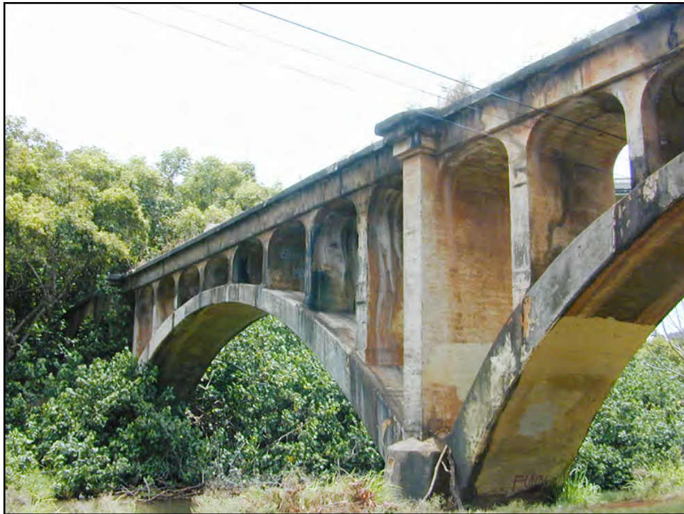
Figure 4b – Photo of the Hanama'ulu Bridge
