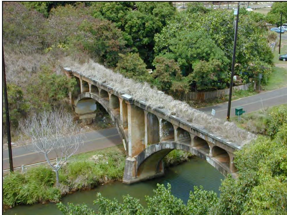
Figure 4a- Photo of the Hanama'ulu Bridge
