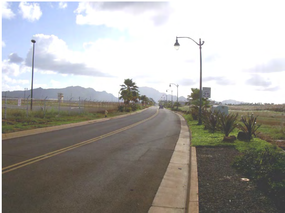
Figure 1b - Improved section of Ahukini Road half way between Ahukini Point and the airport
