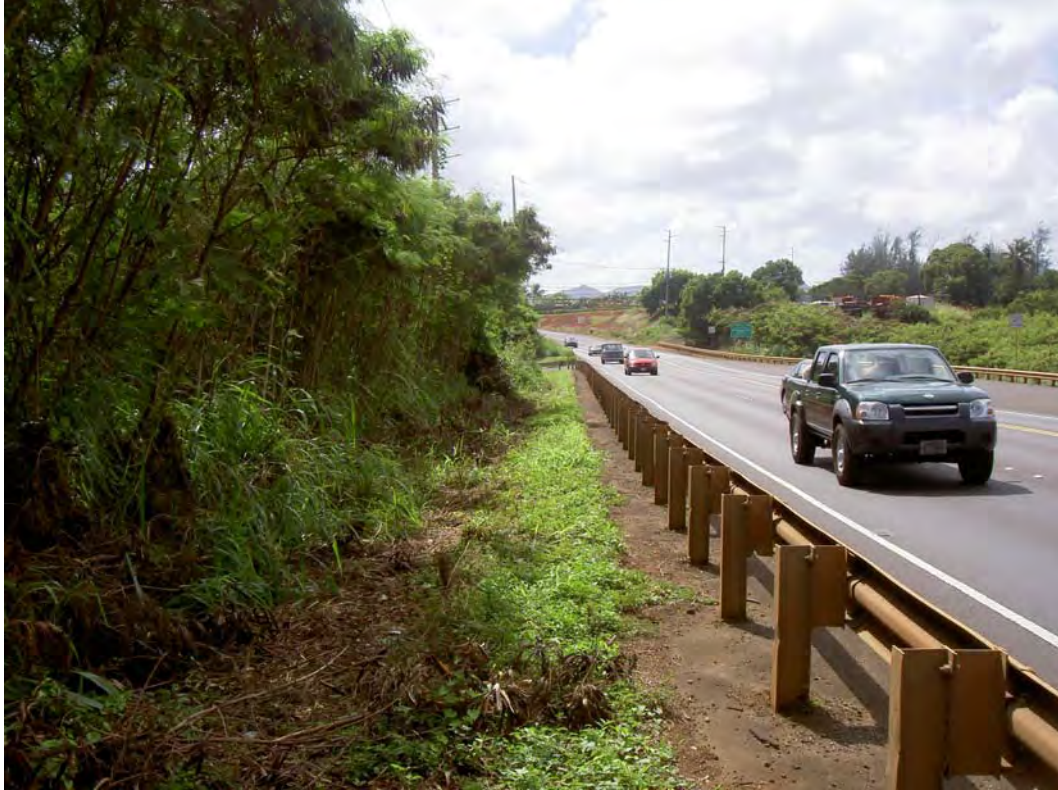
Figure 14c – Photo of area along the highway north of the private business.
