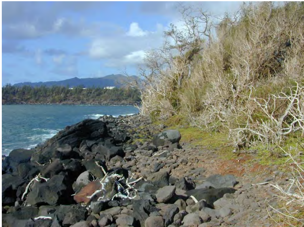
Figure 6b –Photo of the abandoned access road/railroad on the north side of Hanama'ulu Bay
