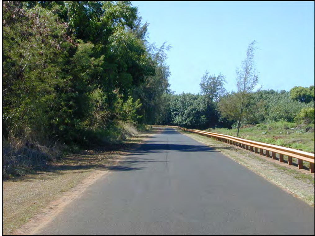
Figure 21b – Photo of Hilton Lane road
