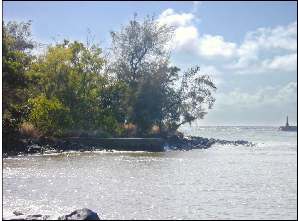
Figure 6a – Photo of Wharf on north edge at Hanama'ulu Bay
