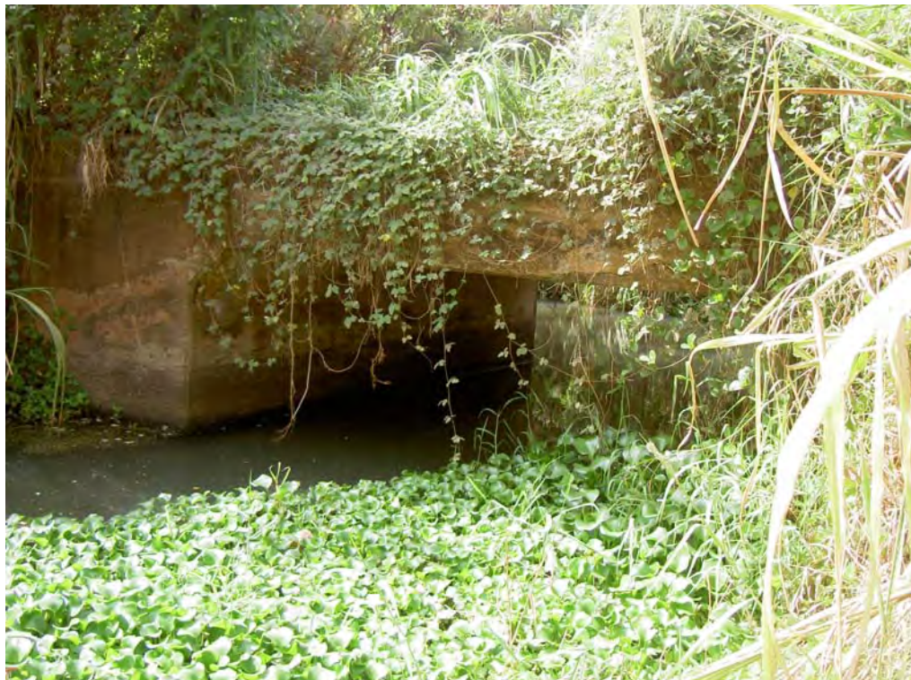
Figure 22b – Photo of the abandoned box culvert railroad bridge
