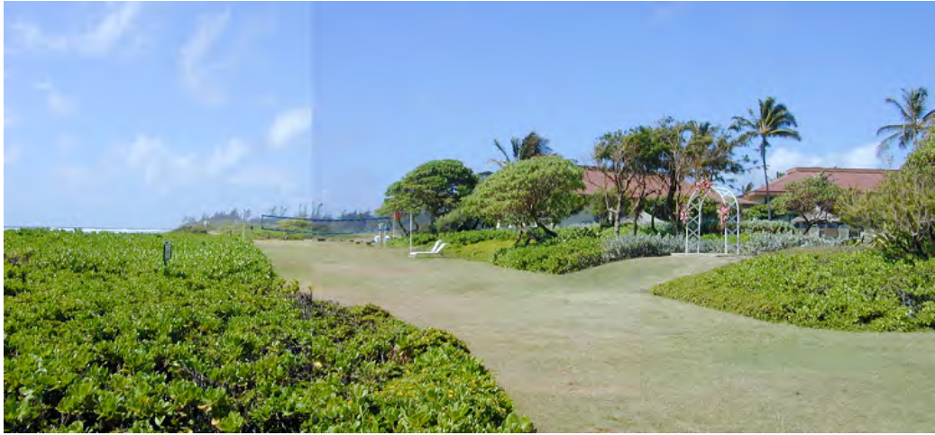
Figure 8b Before photo of the existing shoreline along the Radisson Hotel property
