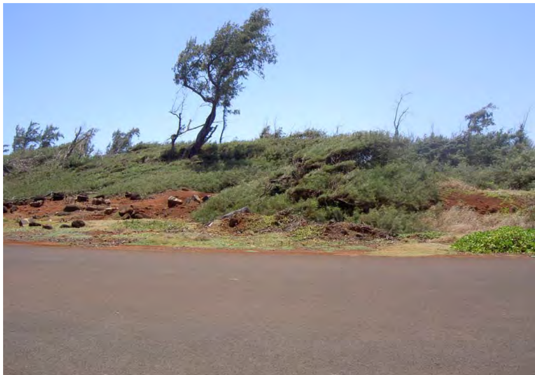
Figure 2b - Photo of the location of the proposed comfort station at Ahukini Point
