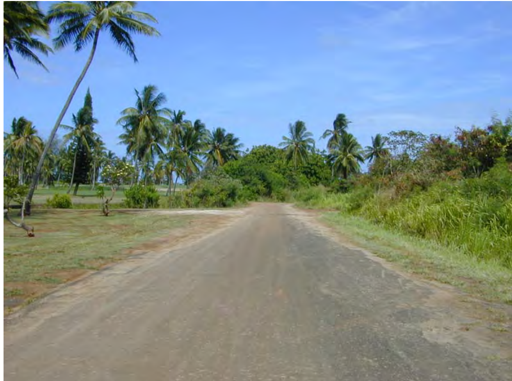
Figure 21a – Photo of un-named cane haul road extending to the Marine Camp site
