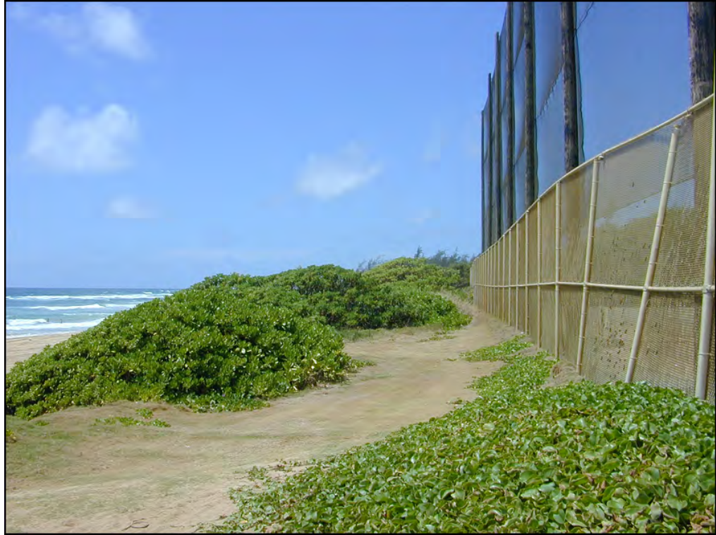
Figure 11g – Photo of the existing conditions behind the driving range fence
