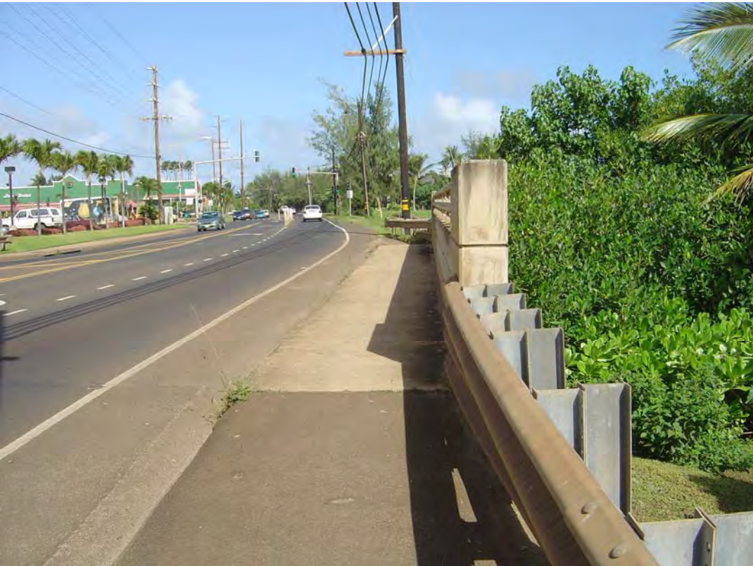
Photo 14. Kuhio Highway at bridge over Uhelekawawa Canal
