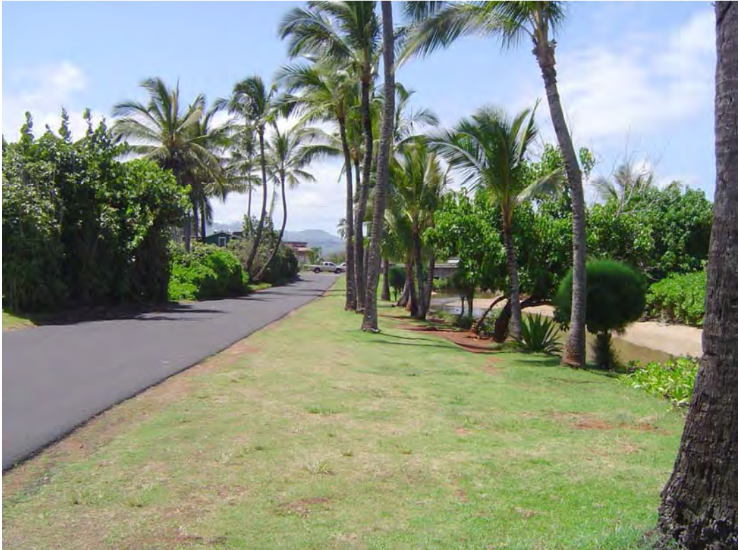
Photo 13. South side of Uhelekawawa Canal
