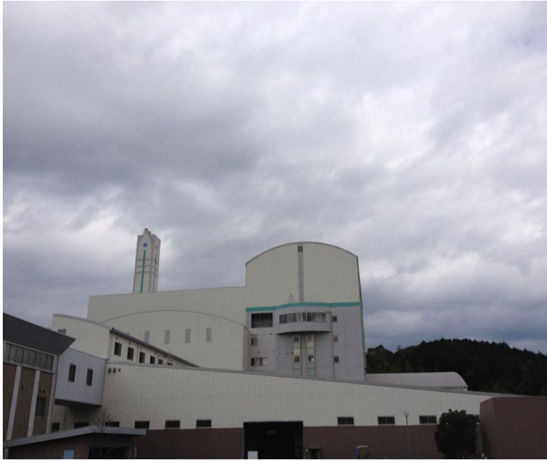
Figure 3: Homan Gasification Plant (Fukuoka, Japan)
