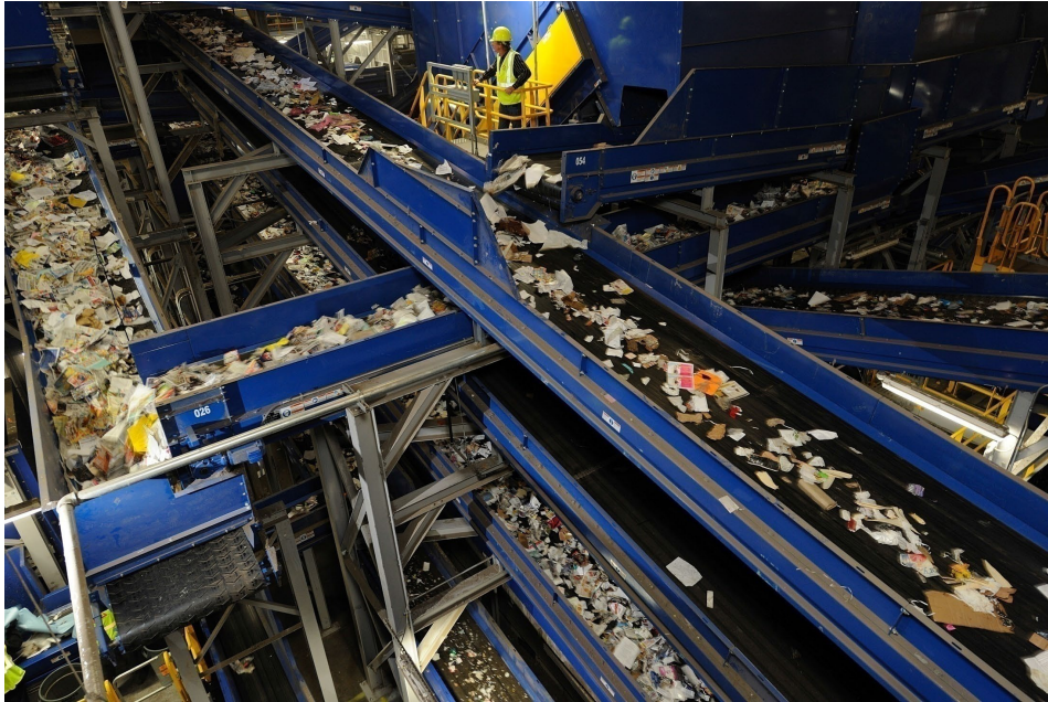
Figure 24: Newby Island Resource Recovery Park, California
