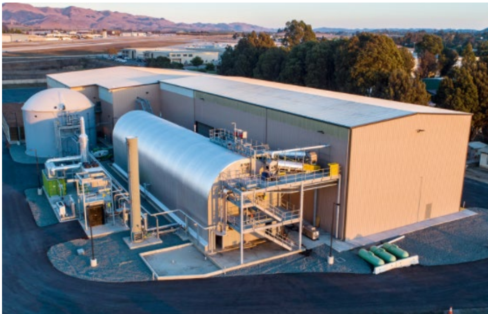
Figure 16: High Solids Horizontal AD Plant, San Luis Obispo, California
