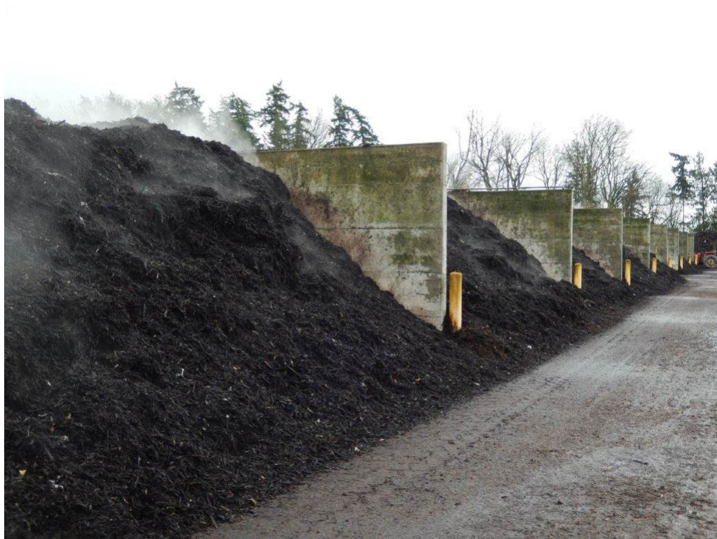
Figure 11: Example of a Bunker Aerobic Static Composting Facility, Stanwood, Washington
